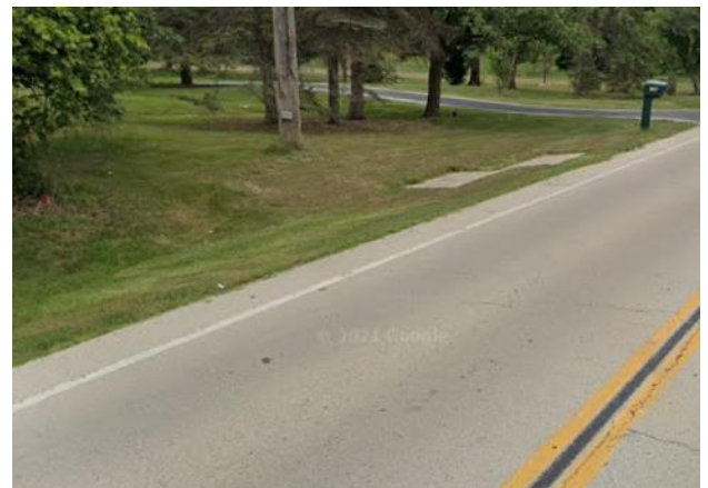
Current open drainage ditch system along Wolf Road.
