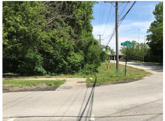
Pedestrian accommodations are not consistently provided along Wolf Road.
